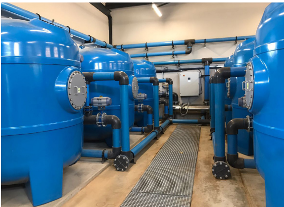
GREY WATER PLANT
