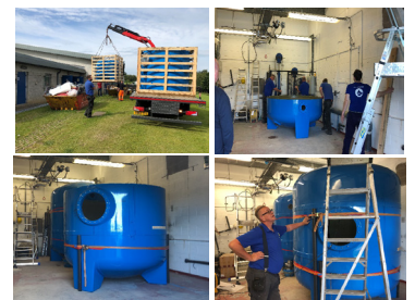
On site assembling
