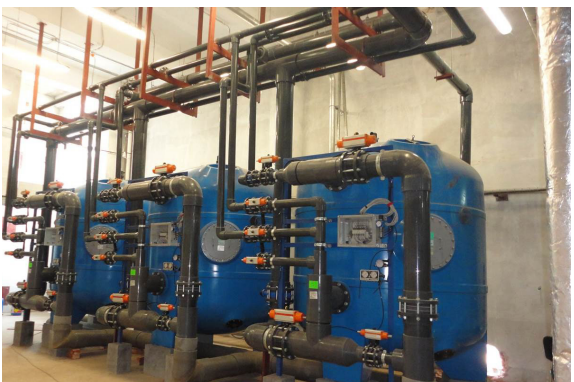
IRON / ARSENIC REMOVAL
