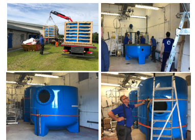
On site assembling
