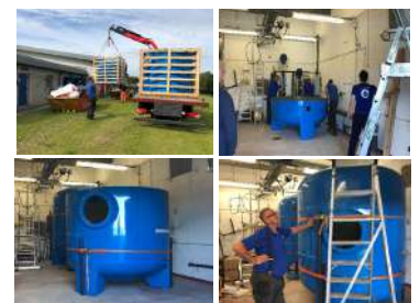
On site assembling
