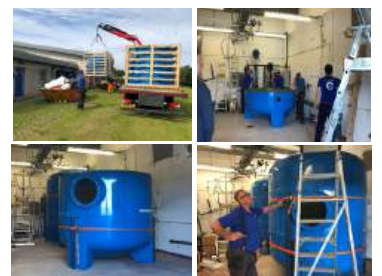
On site assembling
