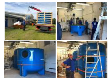
On site assembling
