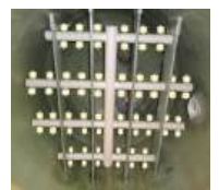
GRP beams with PP nozzles
